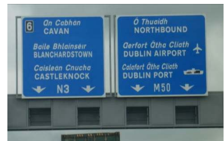
c) Gantry Carrying Directional Signs and Casings for Lane Control Signals, and VMS
