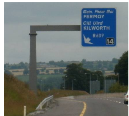
b) Cantilever Gantry
