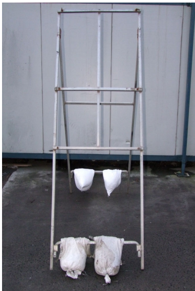
Figure 0.3.2.2.2: Examples of A frames secured with sand bags
