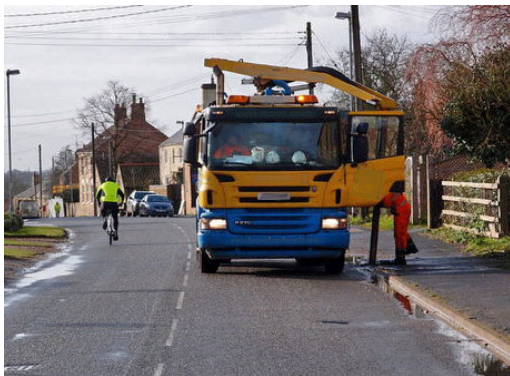
Figure 0.2.2.2.1: Cleaning a blocked gully can be carried out as Type C Works
