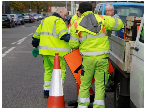
Figure 0.3.2.2.1: Examples of TTM operatives exiting the vehicle on the safe side of the vehicle and a TTM operative working on the wrong side of the vehicle next to live traffic.
