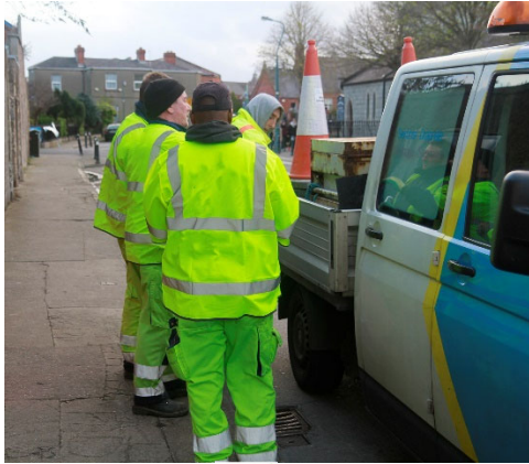
Figure 0.3.2.2.1: Examples of TTM operatives exiting the vehicle on the safe side of the vehicle and a TTM operative working on the wrong side of the vehicle next to live traffic.
