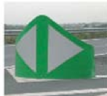
Figure 6.7: Nosing Marker Installation (France)
