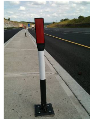
Figure 6.6: Delineator Post at a Lay-by
