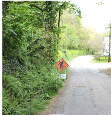
Figure 2.3.3.1: Sign Visibility on Level 2 Roads (cut vegetation around signage)
