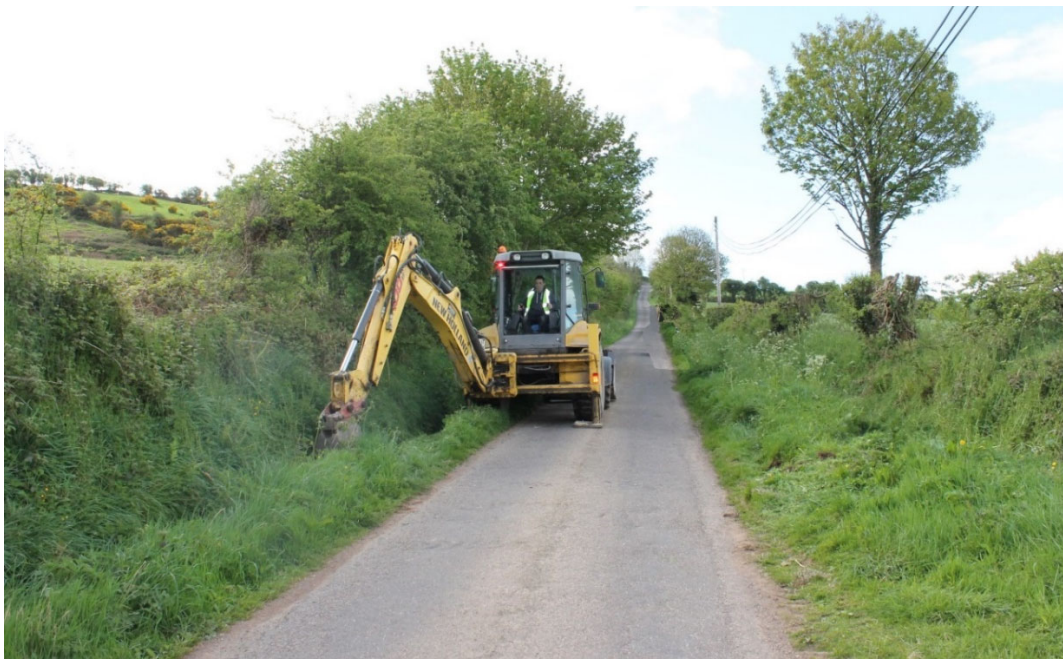
Figure 2.4.4.1: Typical example of Semi-Static Works on a Narrow Road with Unobstructed Road Width < 2.5m. (Semi-Static warning signage has been erected outside of the camera frame)
