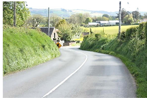
Figure 2.3.3.1: Sign Visibility on Level 2 Roads (cut vegetation around signage)
