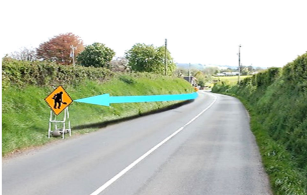
Figure 2.3.3.1: Sign Visibility on Level 2 Roads (cut vegetation around signage)
